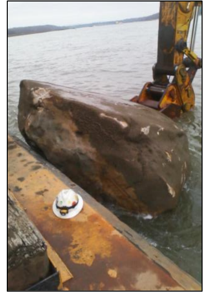
Durocher Rock Removal
